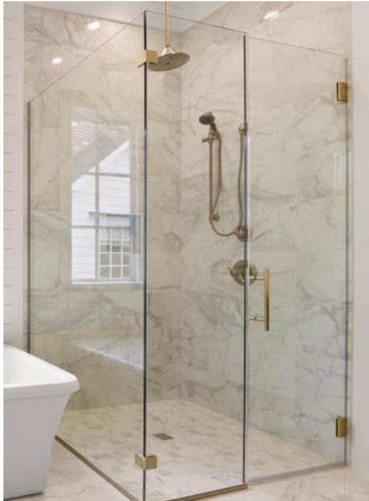
1. **Hinges – Screws on shower door hinges are kept tight.** Over time the action of opening and closing the door will cause the screws to very slowly loosen. Give them an 1/8 to a 1/4 turn once a month to keep them tight. Report any clicking hinges or hinges coming out of the wall immediately to M&M Glass.
